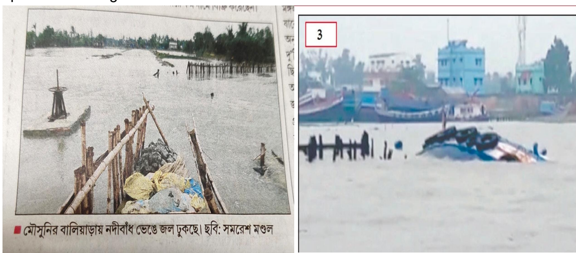
River Barrage at Mousuni Island broken due to impact of Cyclone JAWAD (Anandabazar Patrika dated 06-12-2021)
